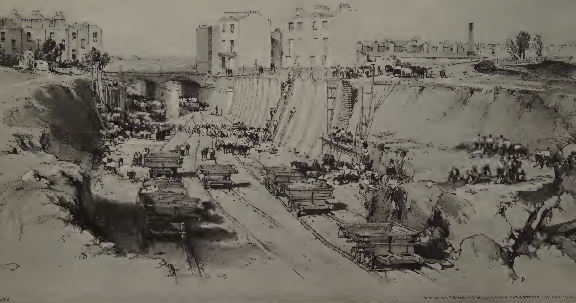
BUILDING RETAINING WALLS NEAR PARK STREET CAMDEN TOWN
