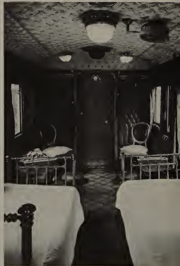
OPPOSITE: The interior of Queen Victoria's private saloon, built in 1869. The furnishings were of yellow satinwood upholstered in royal blue moiré silk, the metal work was of gilt brass, and the walls and ceiling were padded to deaden noise and vibration. BELOW: The Queen's bedroom.
