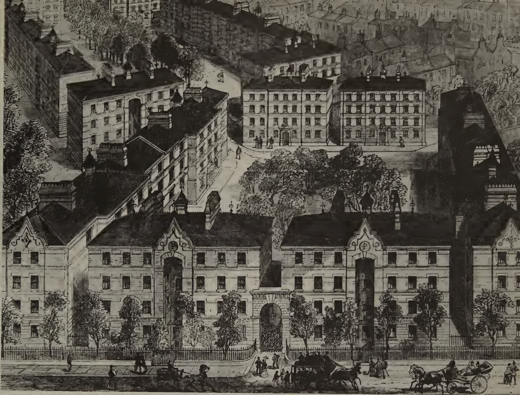
Peabody Square (1871), Blackfriar's Road, a demi-paradise to slum-dwellers re-housed in its trim, if somewhat penitentiary, buildings.
