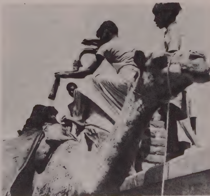
The Djibouti Fire Brigade taking on fresh water
