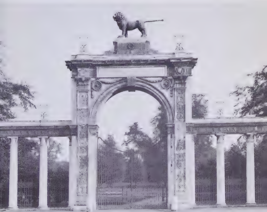
243 Syon House, entrance screen, 1773 (Copyright Country Life )
