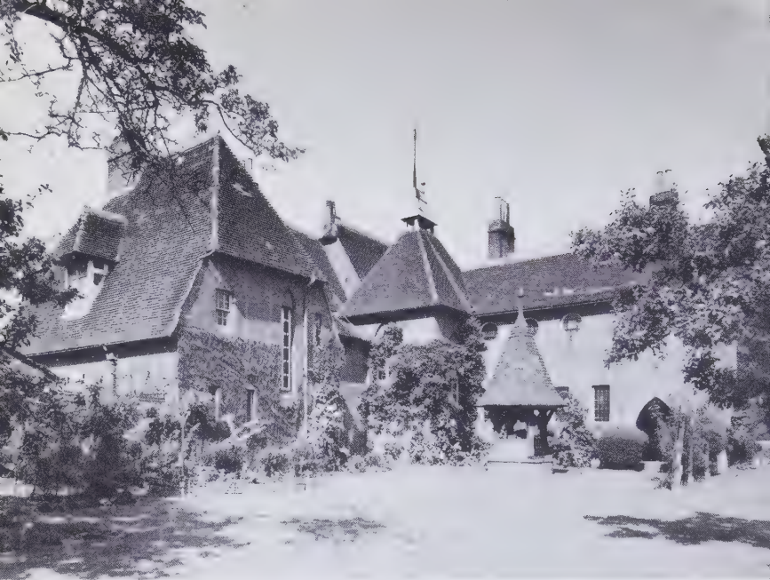
264 Bexley Heath, Kent, Red House, built by Philip Webb for William Morris, 1859
