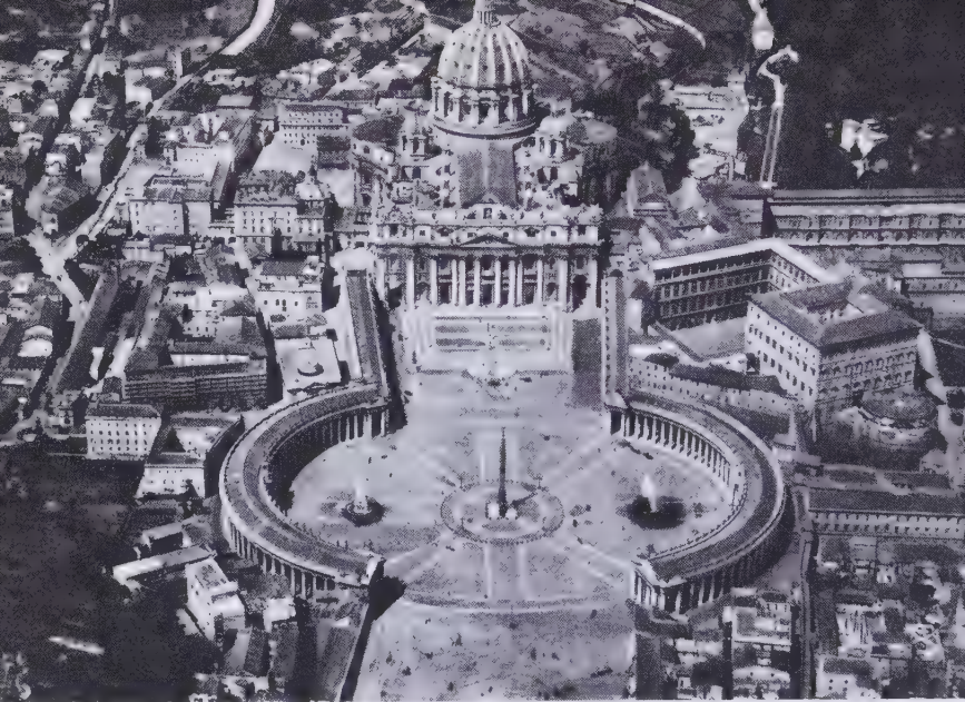
167 Rome, St Peter's Square, with the dome by Michelangelo and della Porta, the front and nave by Maderna, 1607–c.1615, and the colonnades by Bernini, begun 1656
