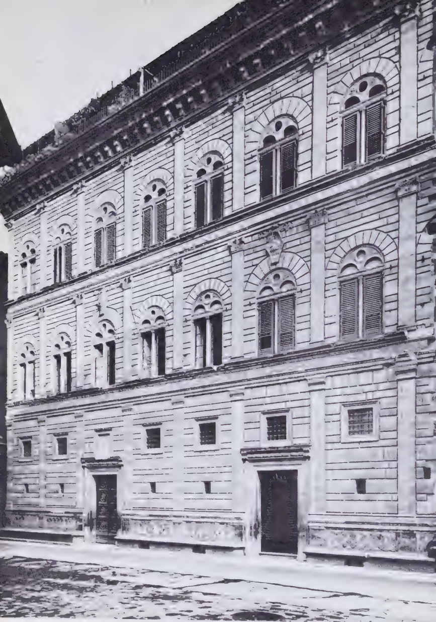
137 Florence, Palazzo Rucellai, by Alberti, built in 1446-51
