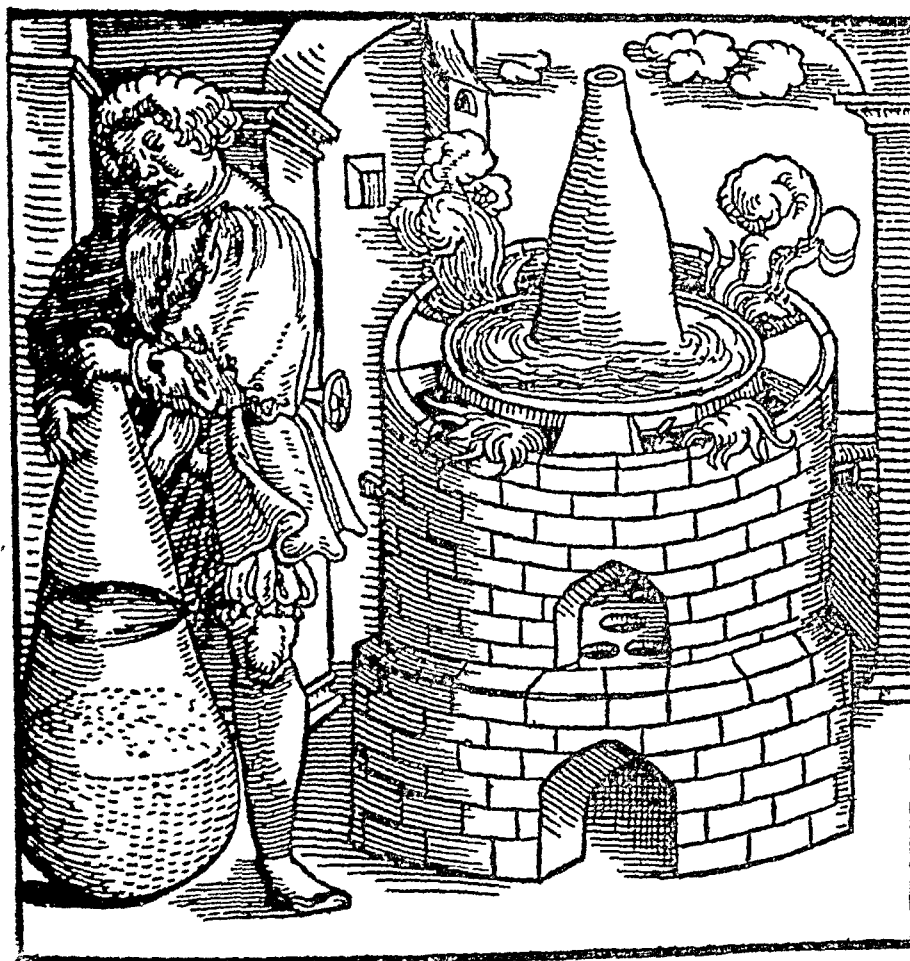
Figure 7 A Water-bath (From The Works of Geber , Englished by R Russell, ed E. J Holmyard, by courtesy of J M Dent & Sons Ltd)
