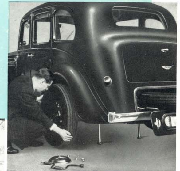
Above A puncture on the road presents little inconvenience to Wolseley owners. The larger models incorporate the built-in Jackall system. The car can be jacked up very simply by operating a small lever from inside the car, and the spare wheel, conveniently situated in a separate compartment at the rear, can be lifted out and changed quickly and easily with the minimum of effort on the part of the driver.
