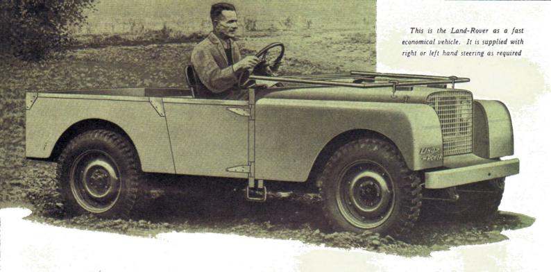
DESIGNED to meet the urgent need for increased production in agriculture and industry, the Land-Rover is a truly multi-purpose vehicle. It is fast and economical for use on the road, and at the same time has that ability to keep going under the very worst cross-country conditions which can only be achieved by four-wheel drive.
