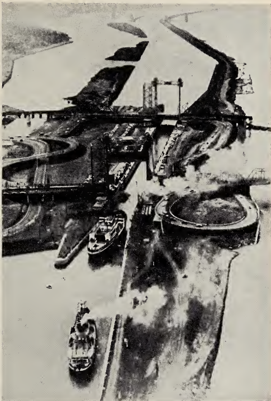
The first ships passed through the St. Lambert Lock into the St. Lawrence Seaway on April 25. The Seaway, which links the St. Lawrence River with the Great Lakes, was officially inaugurated by the Queen and President Eisenhower in the Britannia two months later.
