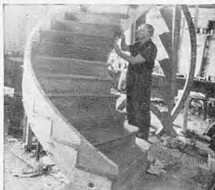
Mr. Foord makes a final adjustment to the curving staircase that he built single-handed in his Eastbourne workshop
