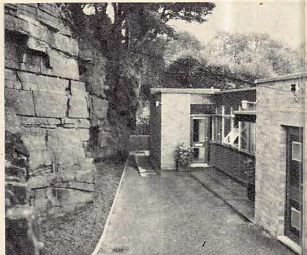
Entrance to Westgate Close, sheltered by rock face. On right is the chamber for the Waterbury gas-fired, blown-air system
