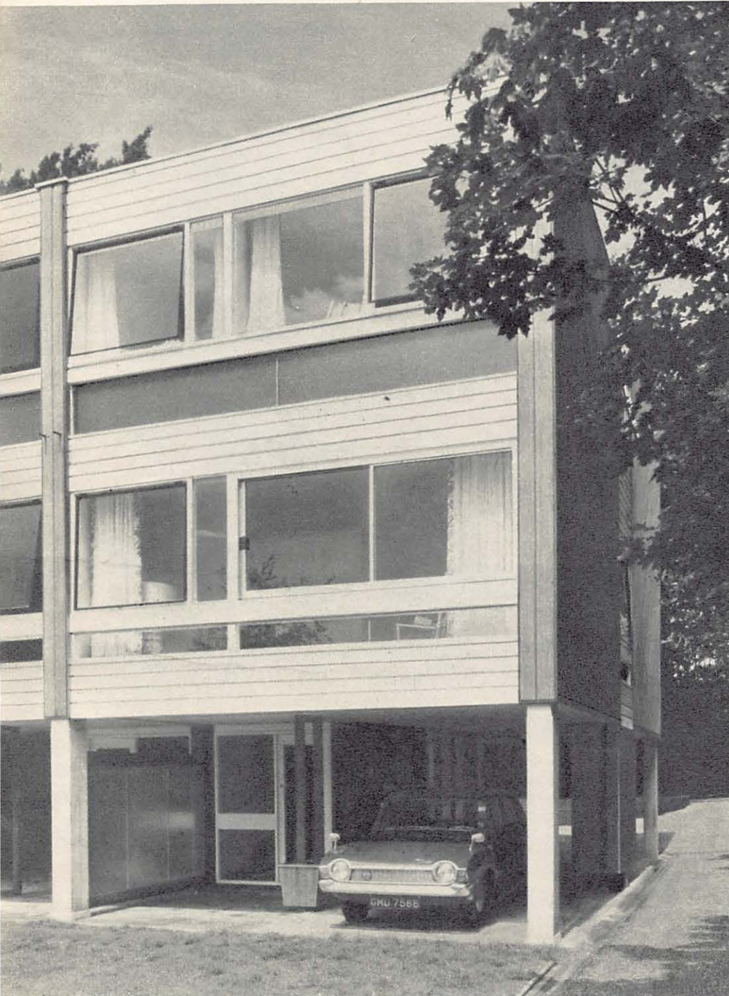
Above, front view of one of the "stilt" houses built in parkland at Beckenham, Kent. Hall, cloakroom, laundry and carport are on the ground floor, with the living areas above and bedrooms on the top floor. The arrangement can be seen in the floor plans shown right. The first-floor plan is the same in all the houses. The top floor can be obtained either with two L-shaped bedrooms, three (as shown) or four with the dressing area converted
