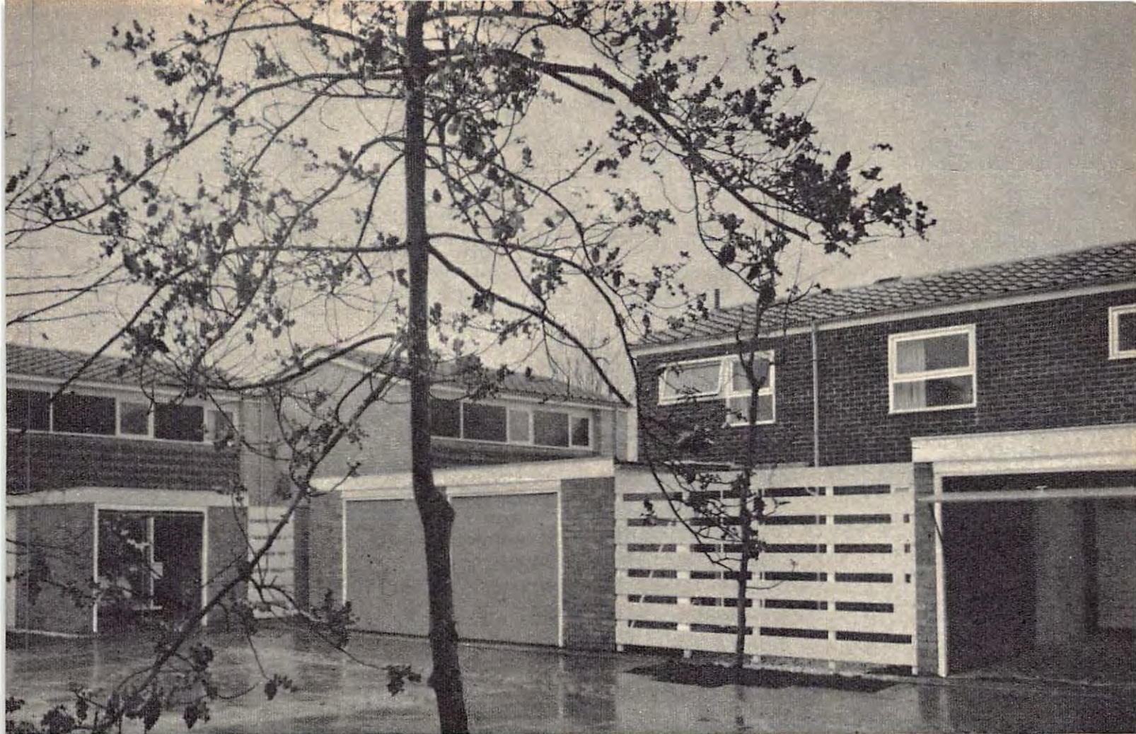
Houses are grouped around the landscaped residential courtyard. Each house has its own private patio, screened by slatted palings
