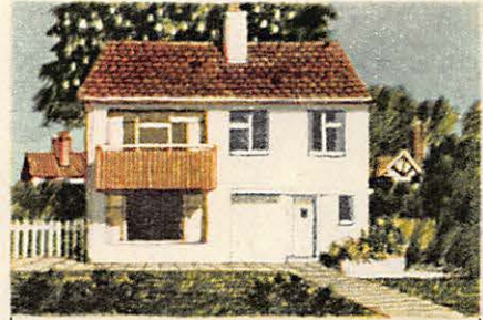
White looks dazzlingly effective on a medium size detached house like this. Cost of Snowcem (2 coats) £6.
