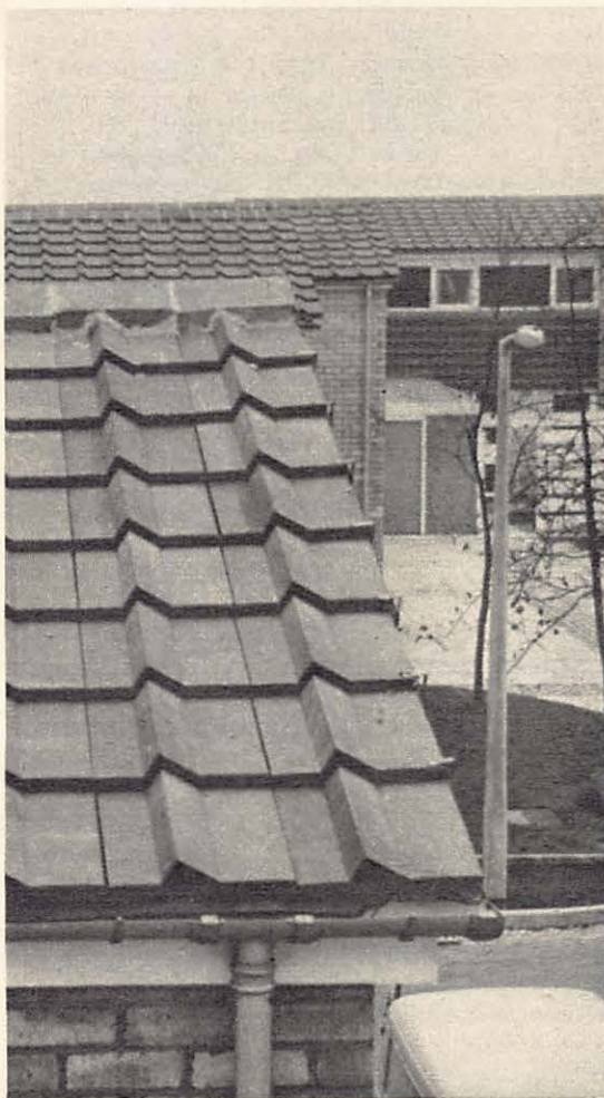
The roofs of the houses at Heaton Norris, Stockport, are of Redland concrete tiles. This is a view from the terrace houses, looking towards the patio homes
