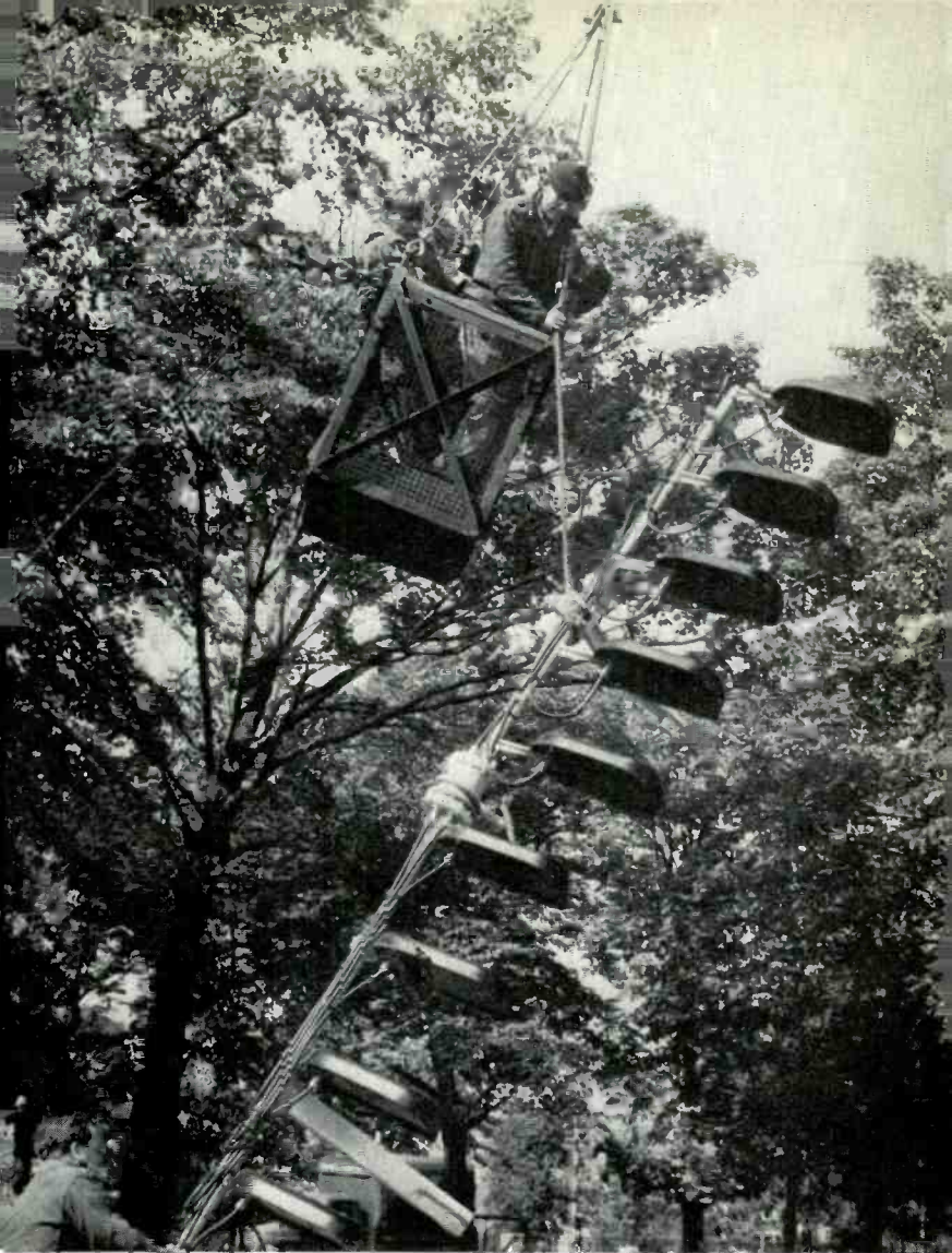
Working at Crystal Palace on the UHF transmitting aerial which will be used for the new BBC-2 625-line UHF transmissions
