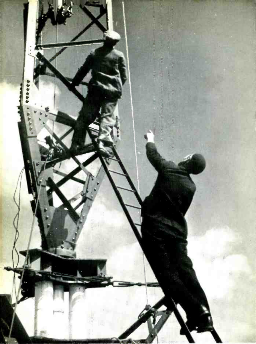
Erecting the first mast at the new Start Point Transmitting Station
