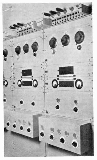
THE CONTROL ROOM AT BROADCASTING HOUSE TWO OF THE RECEIVERS USED FOR CHECKING THE QUALITY OF TRANSMISSIONS
