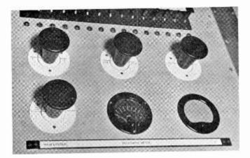
THE CONTROL ROOM IN BROADCASTING HOUSE DETAILS OF A CONTROL POSITION, SHOWING A FOUR-CHANNEL FADE UNIT
