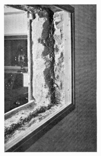
EEL GRASS FOR SOUND-INSULATION SANDWICHED IN WALLS OF PUMICE CONCRETE
