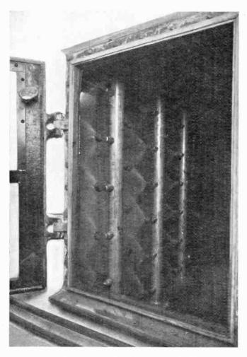
AIR-CONDITIONING PLANT. THE WATER SPRAY FOR WASHING SOOT AND DUST FROM THE AIR DRAWN IN FROM THE STREET
