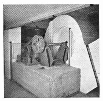
ONE OF THE FANS AND FAN MOTORS OF THE AIR-CONDITIONING EQUIPMENT FOR THE CONCERT HALL Note the massive vibration-insulating joint
